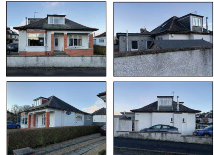
03 Existing Photos Scale NTS @ A1
