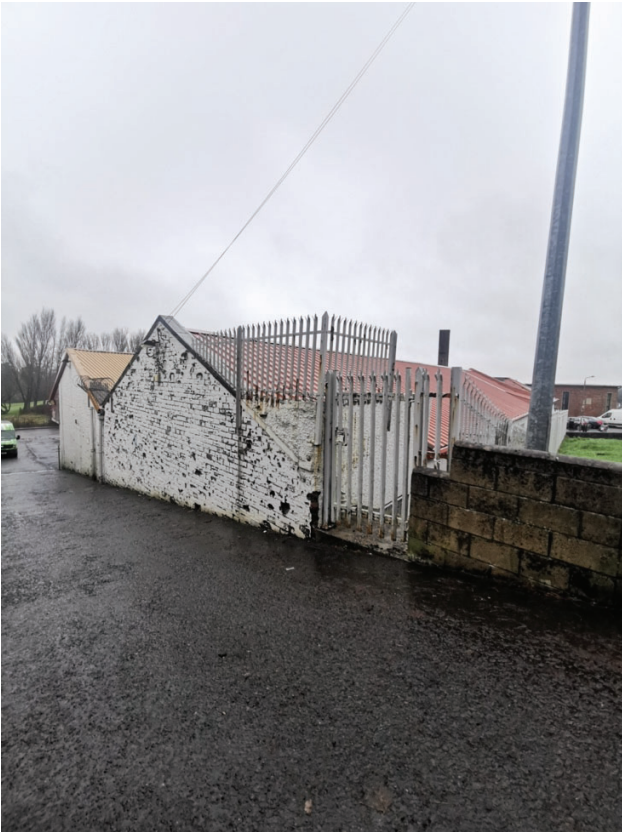
Existing warehouses on site viewed from Stamperland lane.
