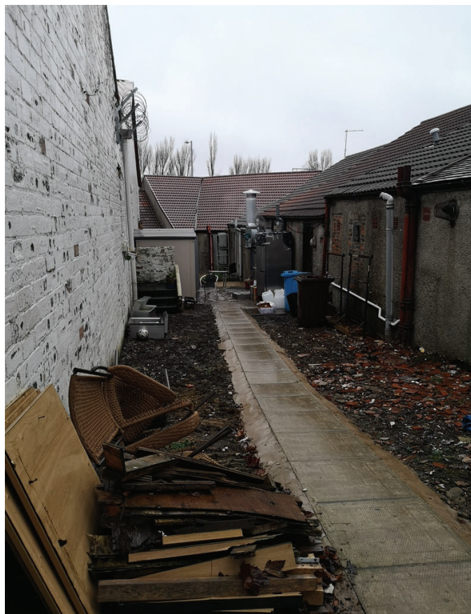
Photo of the condition to the rear of the shops
