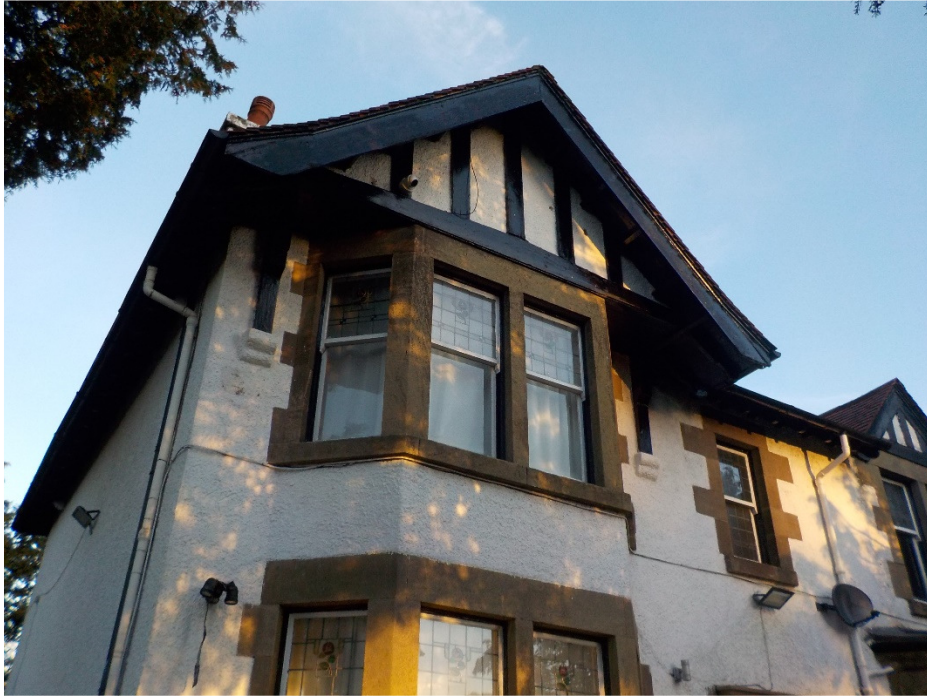
Photograph No.5 – Front left-hand, first floor bay window
