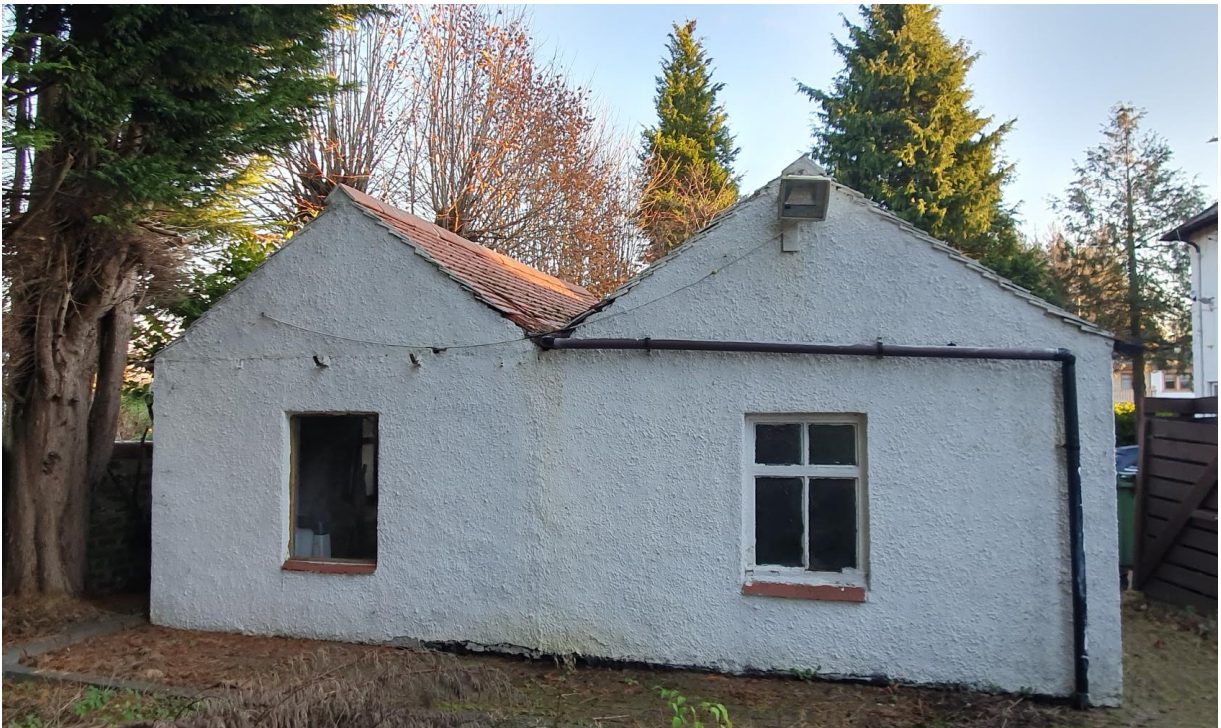
Plate 6. Garage from northwest (rear)
