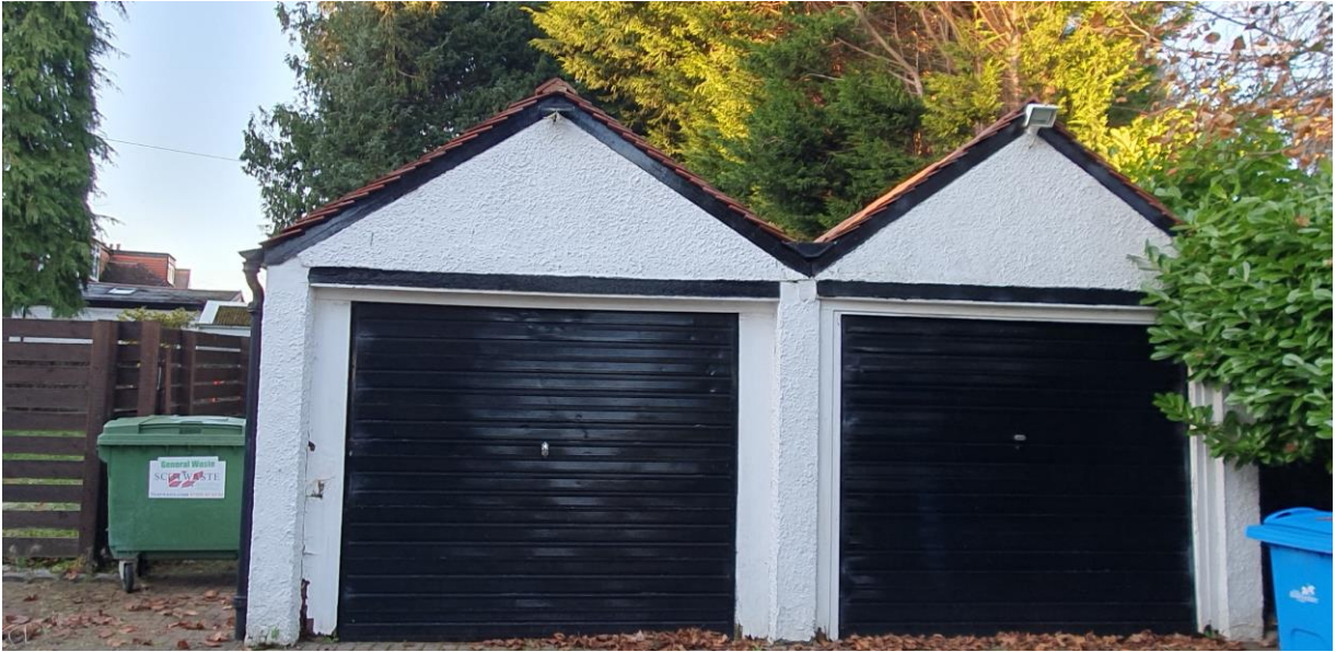
Plate 5. Garage externals from southeast (frontage)
