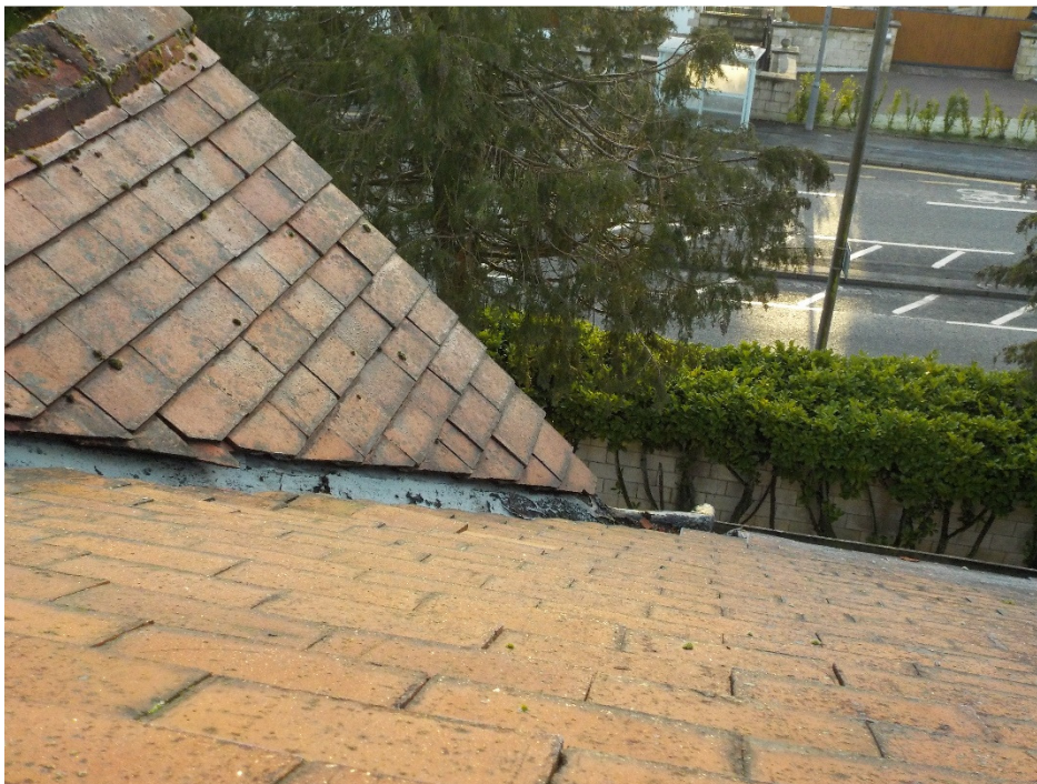
Photograph No.18 – View of valley gutter on front side of roof
