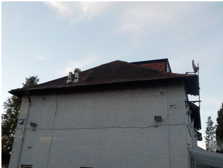
Photograph No.14 – Right-hand gable elevation
