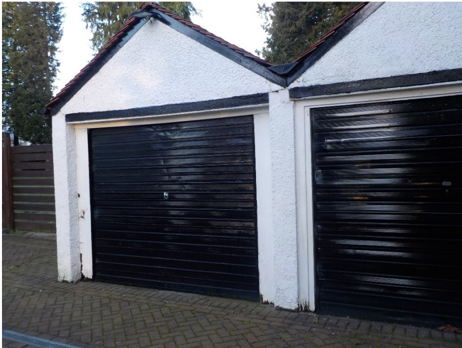
Photograph No.22 - Front elevation of garage
