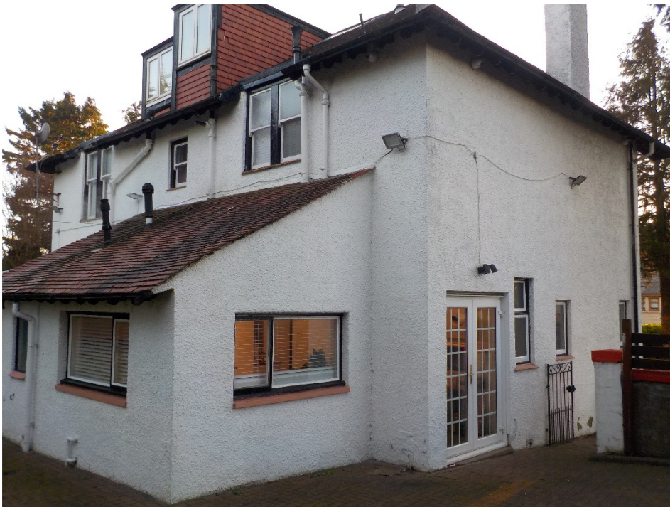
Photograph No.8 – Rear/left-hand gable elevation
