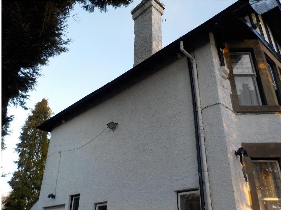
Photograph No.7 – Left-hand gable elevation
