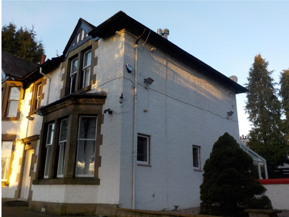
Photograph No.13 – Right-hand gable elevation
