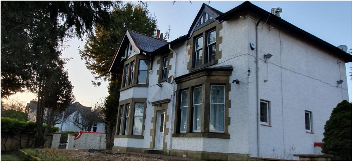
Plate 1. Frontage of dwellinghouse from east
