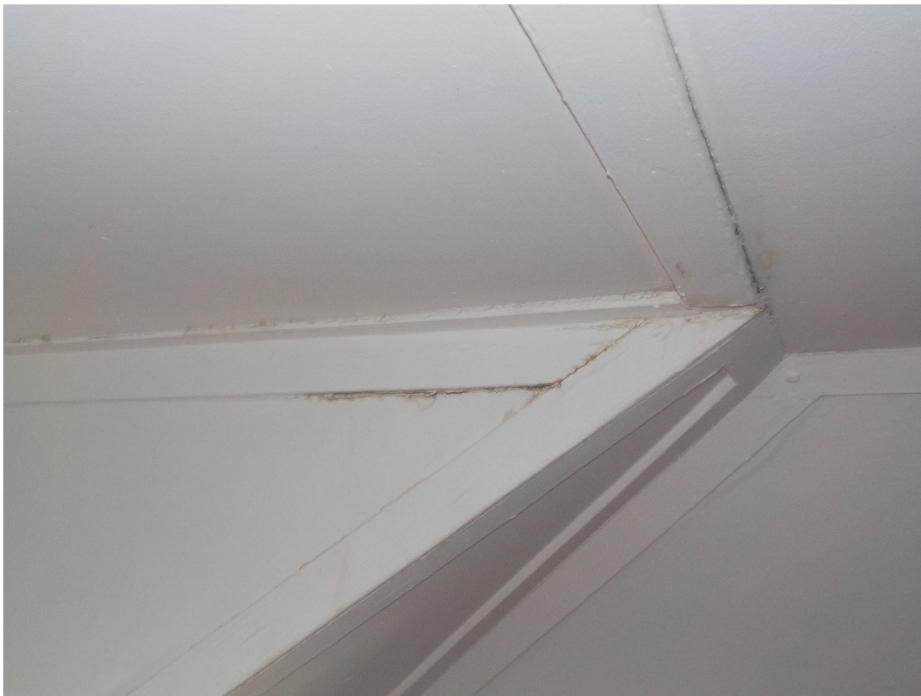
Photograph No.20 – As Photo 19.
