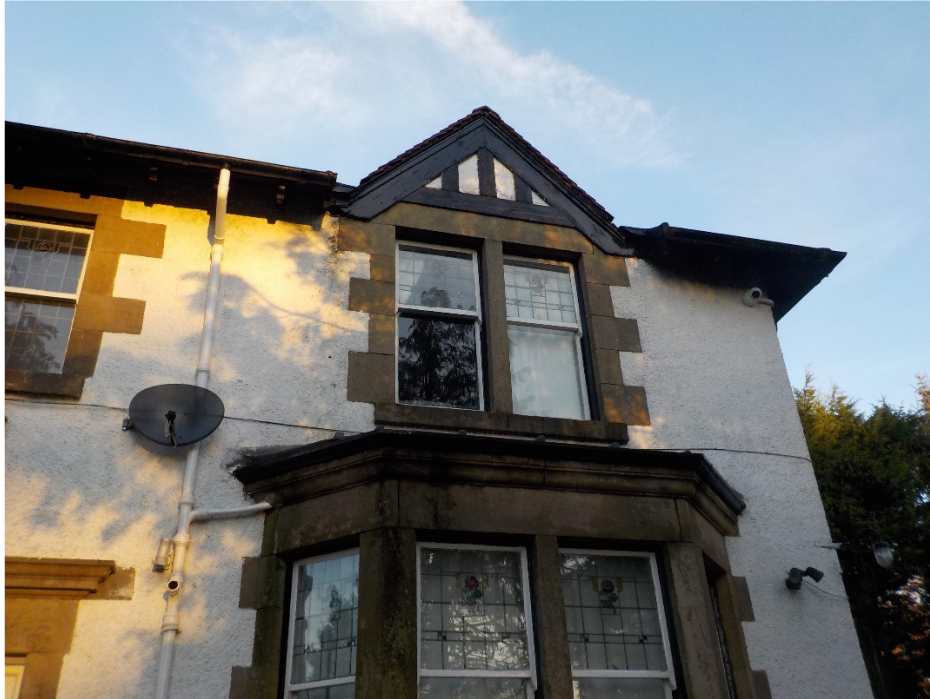
Photograph No.3 – Front right-hand first floor window
