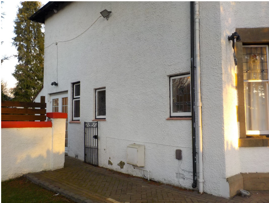
Photograph No.6 – Left-hand gable elevation
