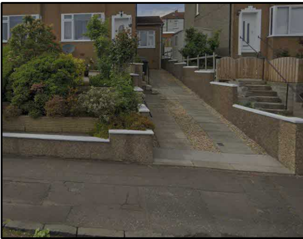
Non roads compliant example within area showing fencing, masonry etc. Elevated to similar level as proposal
