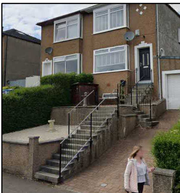
Non roads compliant example within area. Elevated to similar level as proposal
