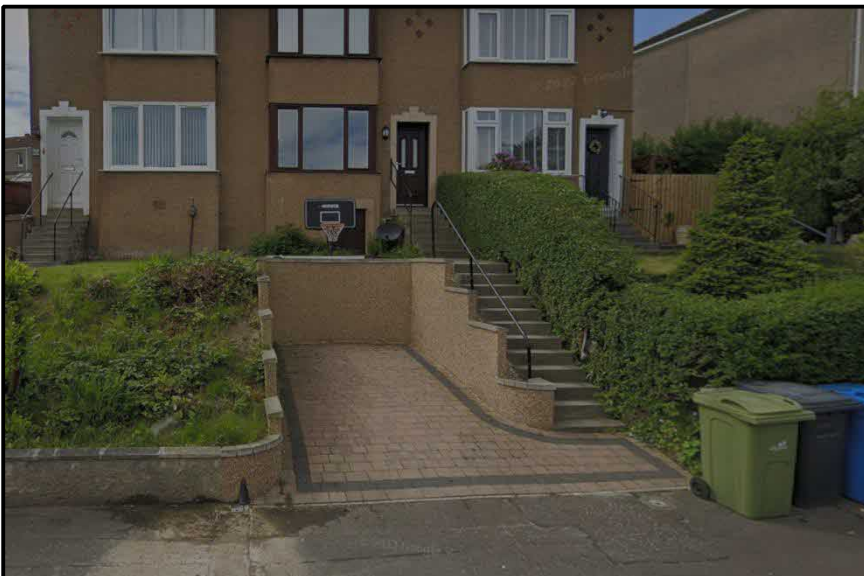
Constructed front driveway again with steps to front of house.
