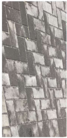
New Permeable Paving
