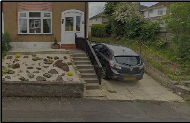
Non roads compliant example within area showing fencing, masonry etc. Elevated to similar level as proposal
