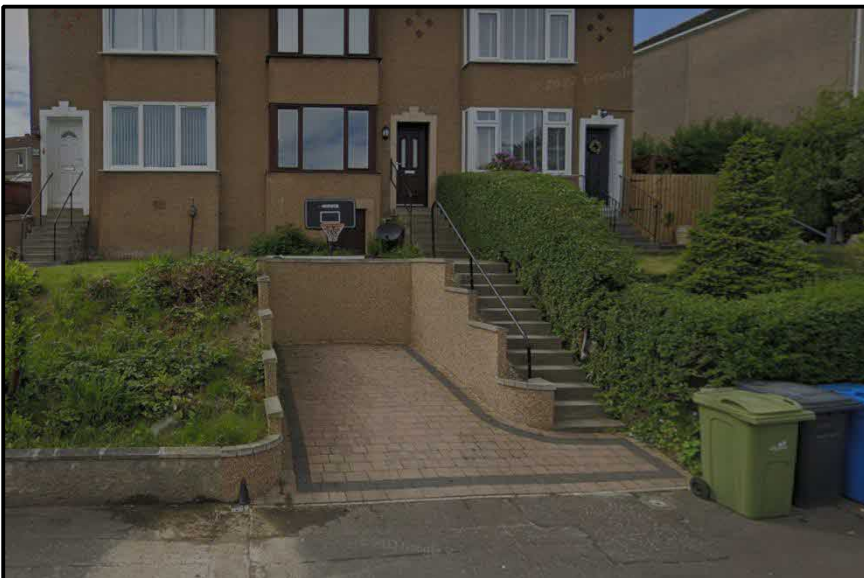
Constructed front driveway again with steps to front of house. Elevated to similar level as proposal
