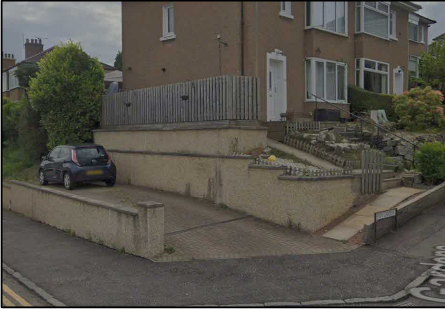
Non Roads compliant driveway however example of streetscape with walls, fencing etc, door. Elevated to similar level as proposal
