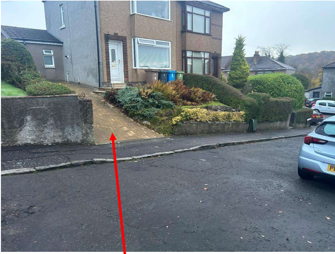
Wall preventing inter pedestrian visibility & Gradient to steep.
