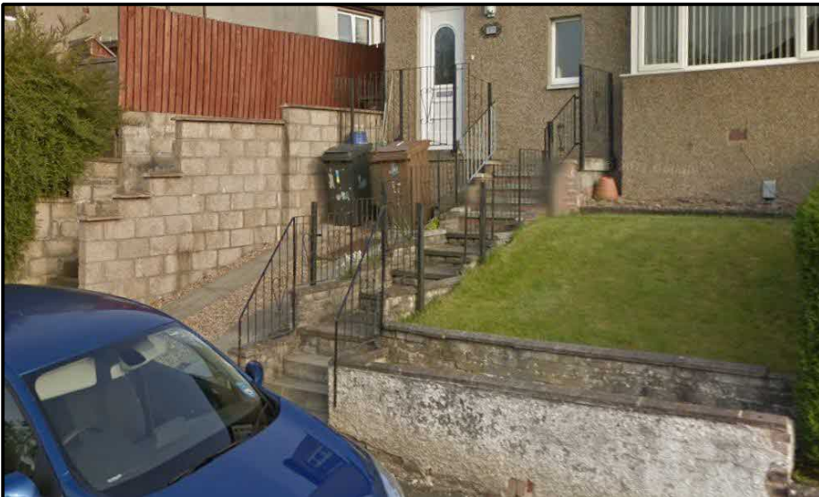
Example of handrails, retaining walls, fencing and hard landscaping within the area. Elevated to similar level as proposal
