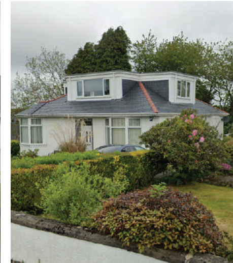
1 Gilmourton Crescent, G77 5AE Adjoining dormers, meeting the existing roof hip and ridge.
