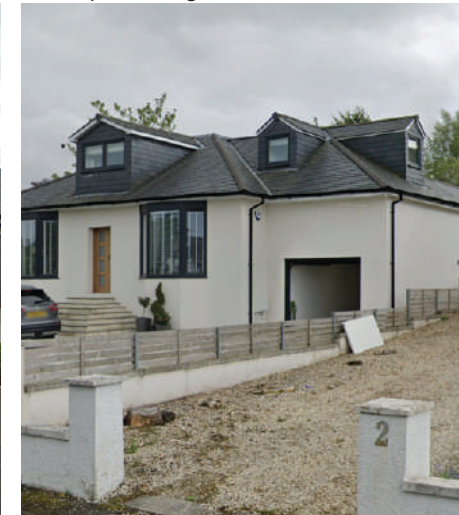
4 Ford Road, G77 5AB Adjoining dormers, meeting the existing roof hip and ridge.
