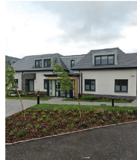
52 Eaglesham Road, G76 7TP Building off of wall head.
