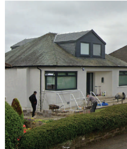
48 Paidmyre Road, G77 5AJ Meeting the existing roof hip and ridge.
