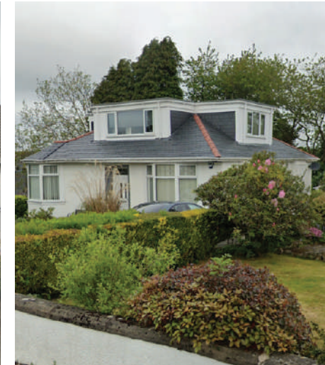
1 Gilmourton Crescent, G77 5AE Adjoining dormers, meeting the existing roof hip and ridge.
