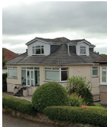
52 Paidmyre Road, G77 5AJ Meeting the existing roof hip and ridge.
