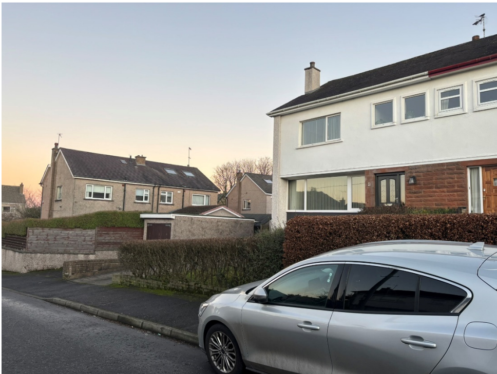
The rear dormer will also not be visible from Kippen Drive as per the photo above. This photo shows the rear elevations of numbers 92 and 94 East Kilbride Road from this approach. The proposed rear dormer will only be visible from the rear gardens of the lower odd numbers of Kippen Drive.
