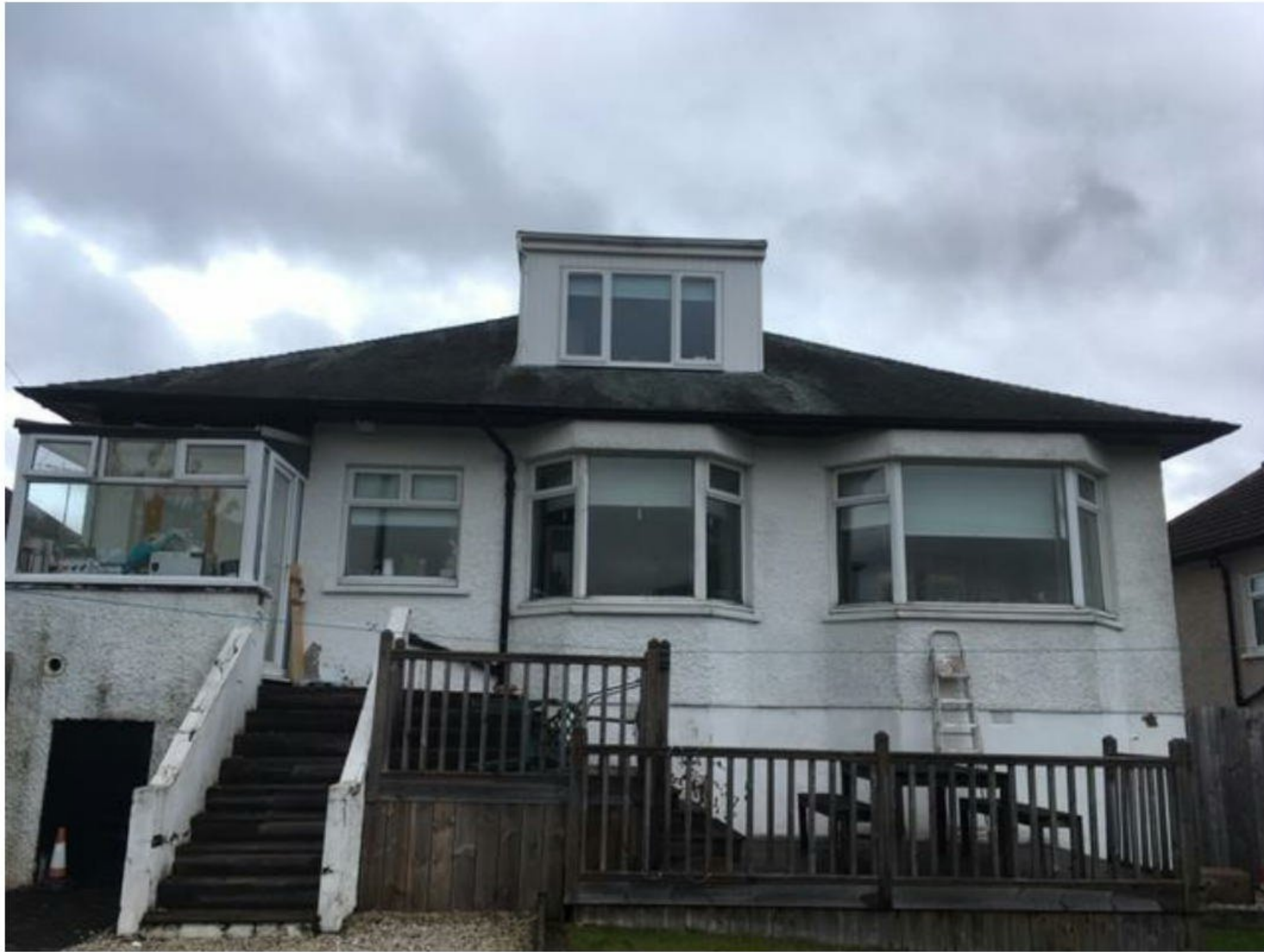
Figure NPD2: Image of Rear Elevation of 48 Paidmyre Road
