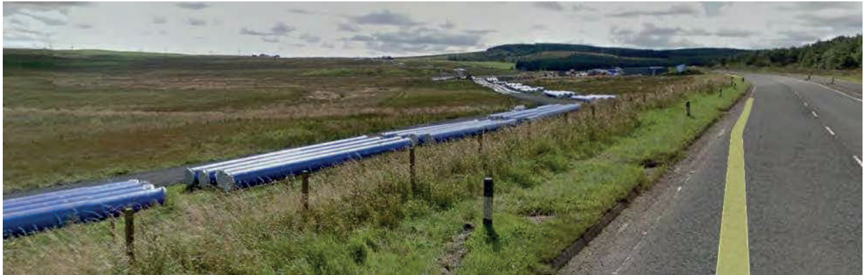
Figure 2.2: Scottish Water's Works
