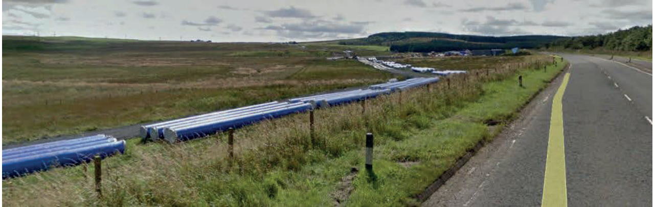
Figure 2.2: Scottish Water's Works
