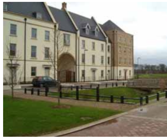
In Upton, Northamptonshire, convenient pedestrian links have been created to allow pedestrians a quick route across the swale.
