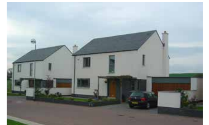
Villas with integrally designed walling create a unified street
