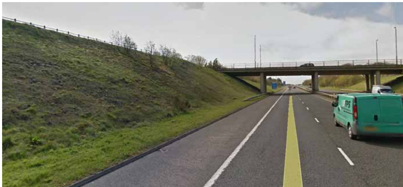
Topography Site 1 - M77 Cutting at the Western Edge of the Site
