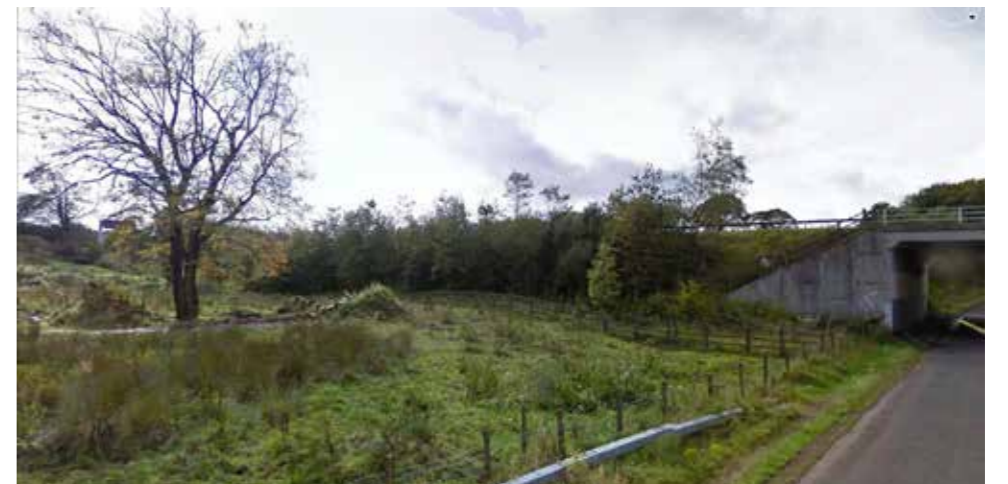
Low northern area at Netherplace Road with M77 Bridge
