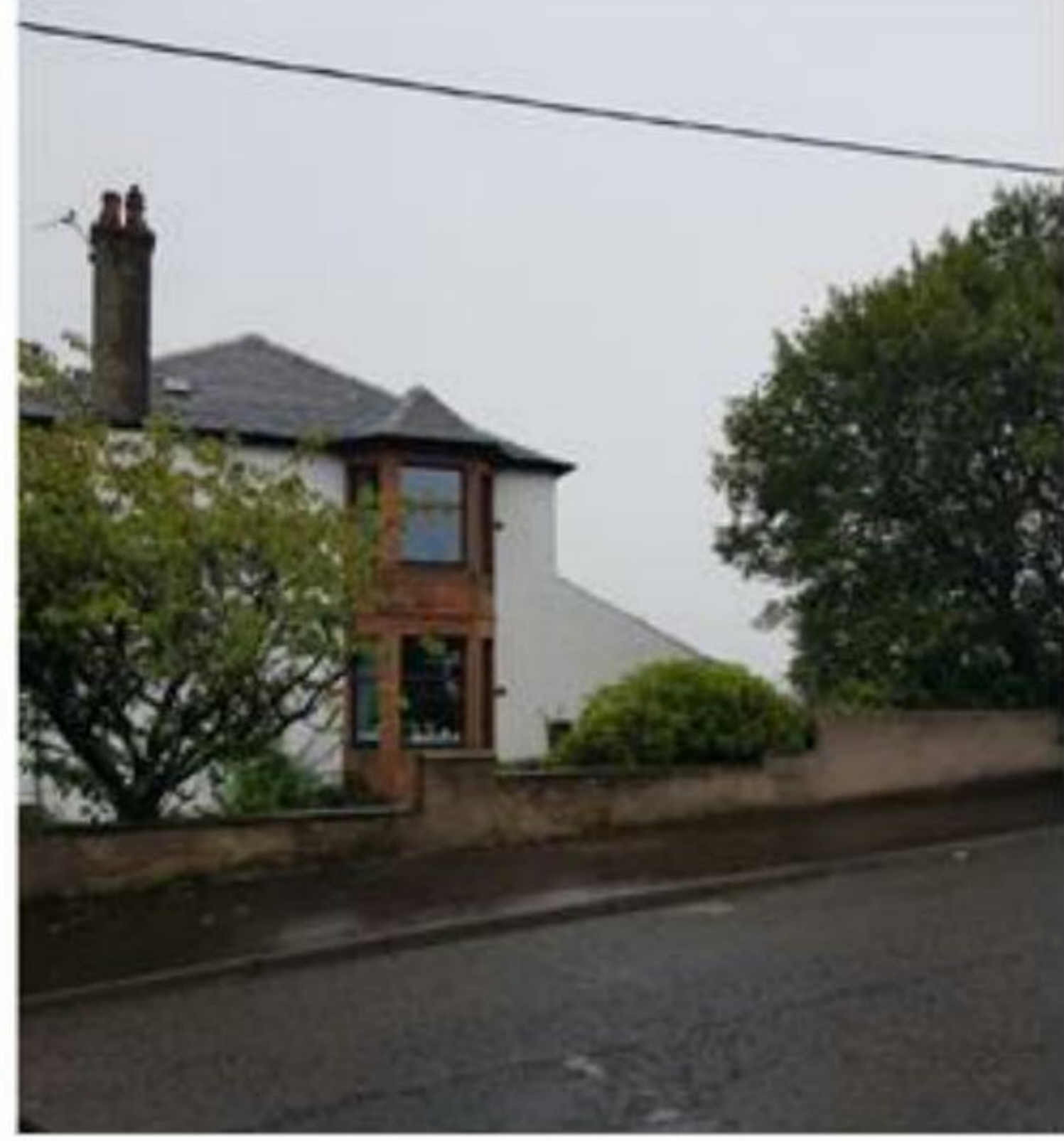
View from Church Road illustrating change in levels across site boundary
