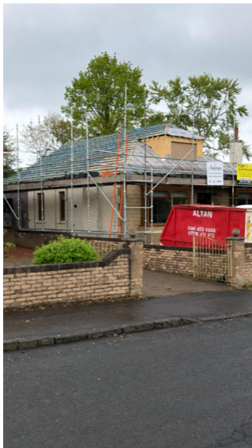
Extension now currently in progress for Evan Drive
