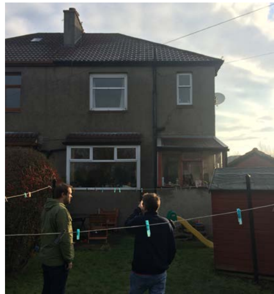
Figure 3: Existing rear elevation
