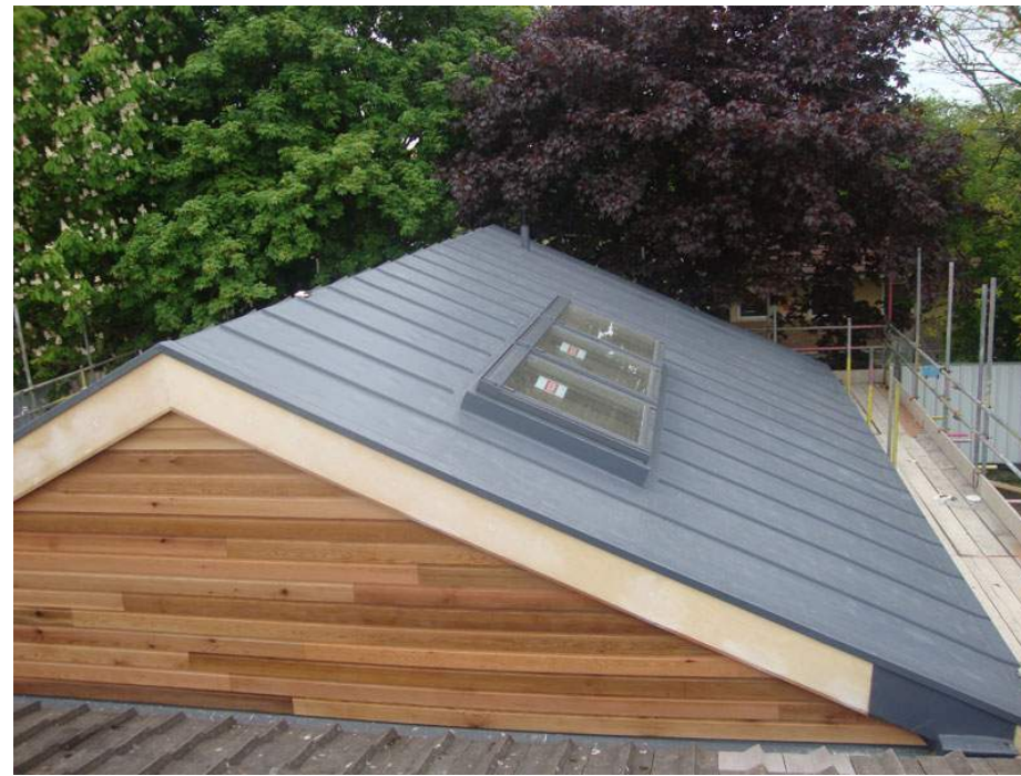
Roofing membrane with raised seams
