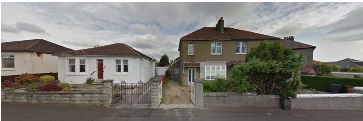
Figure 1a: Housing on Balmeg Avenue, Giffnock
