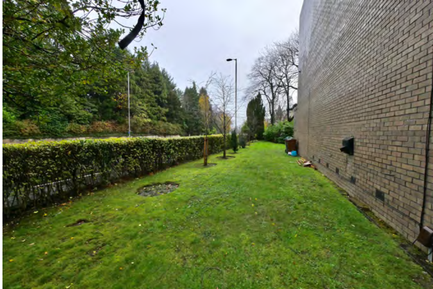
Site photograph indication hedge, missing tree and saturated grass.
