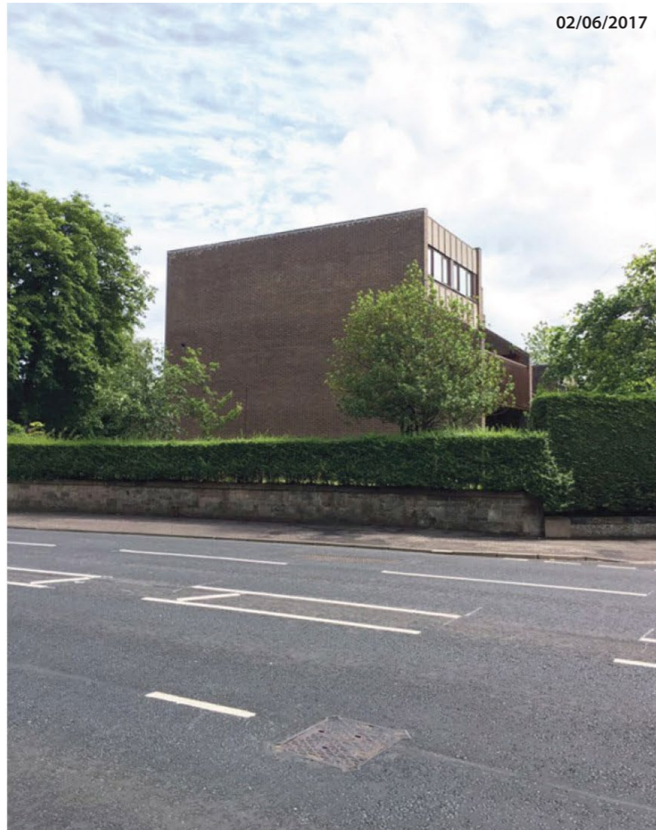
1. Note height of hedge on right corner. Beech hedge to its left would be allowed managed growth to match this.
