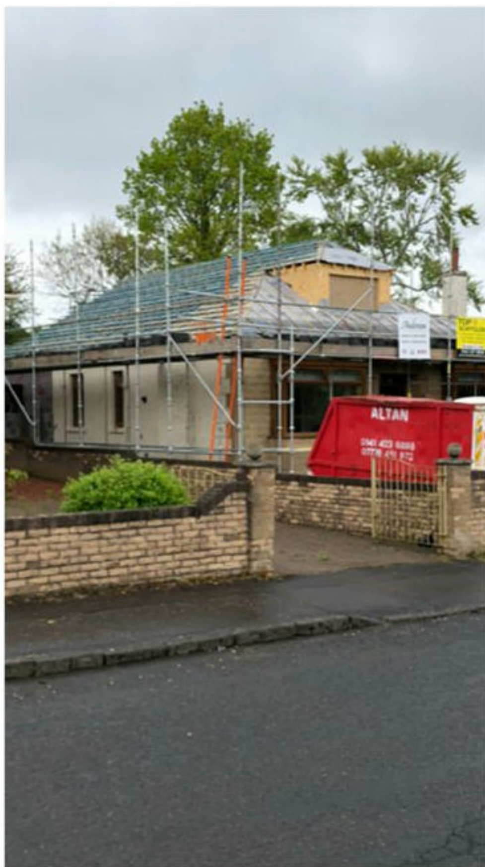
Fig 7 Extension now currently in progress for Evan Drive
