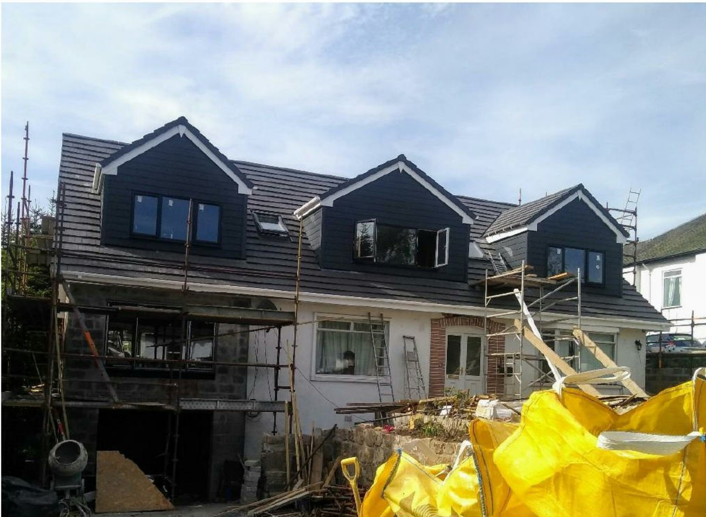
Image # 2: 3 Craigie Drive remodel nearing completion
