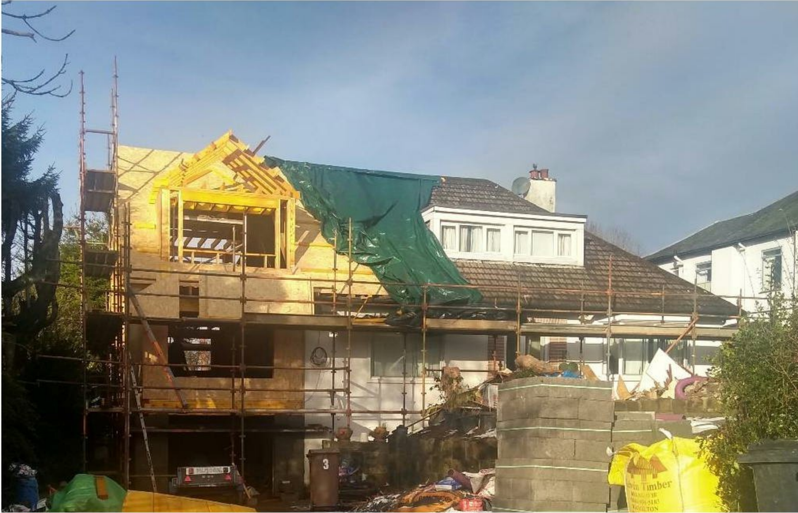
Image # 1: 3 Craigie Drive remodel in progress
