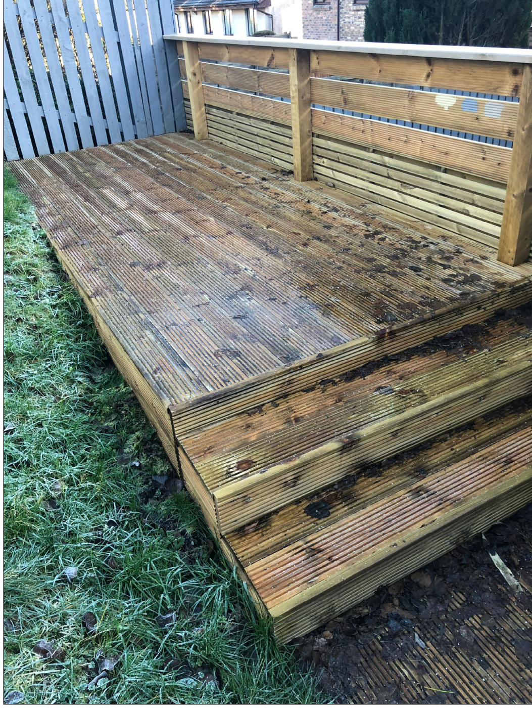
AS BUILT TERRACE PHOTO 1
