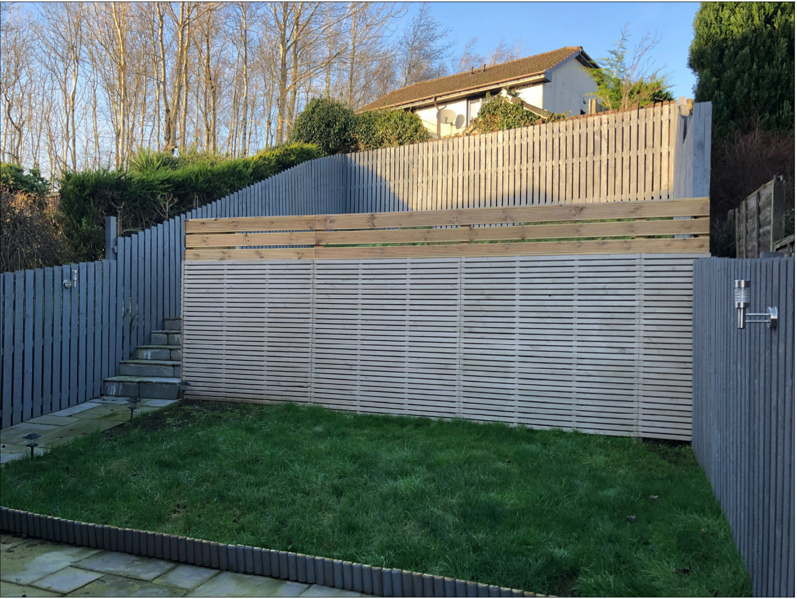
AS BUILT TERRACE PHOTO 2
