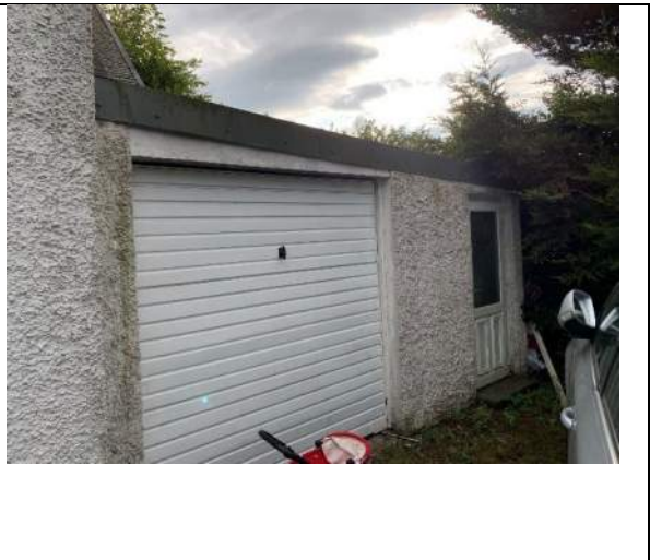
Plate 4 – North elevation garage
