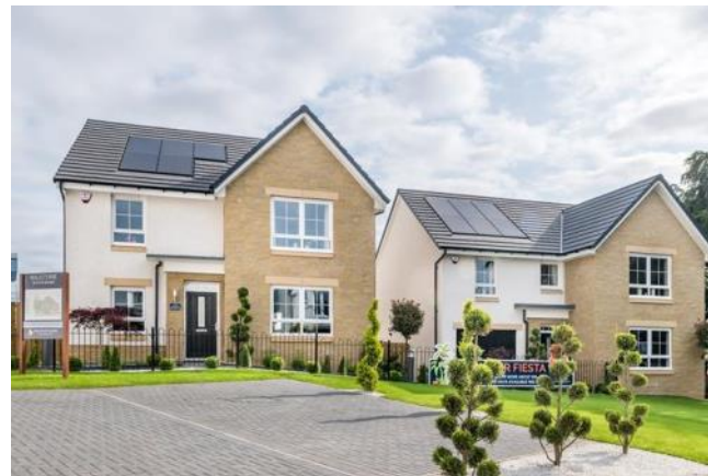
Recently completed 2 Storey Houses (neighbouring Barratt Homes site to west)
