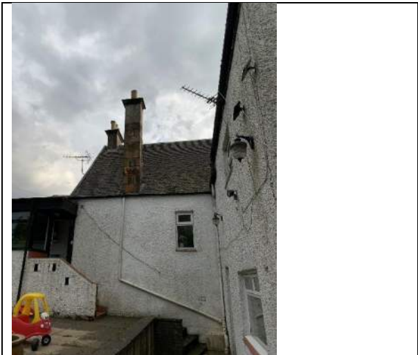
Plate 3 – North elevation of cottage
