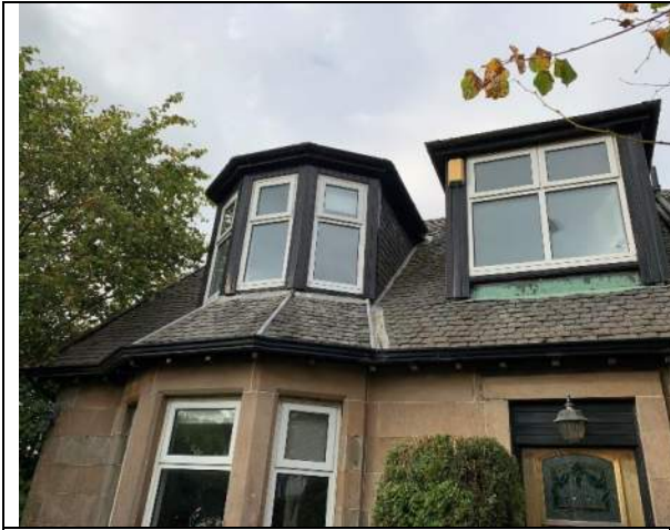
Plate 1 – South elevation of cottage
