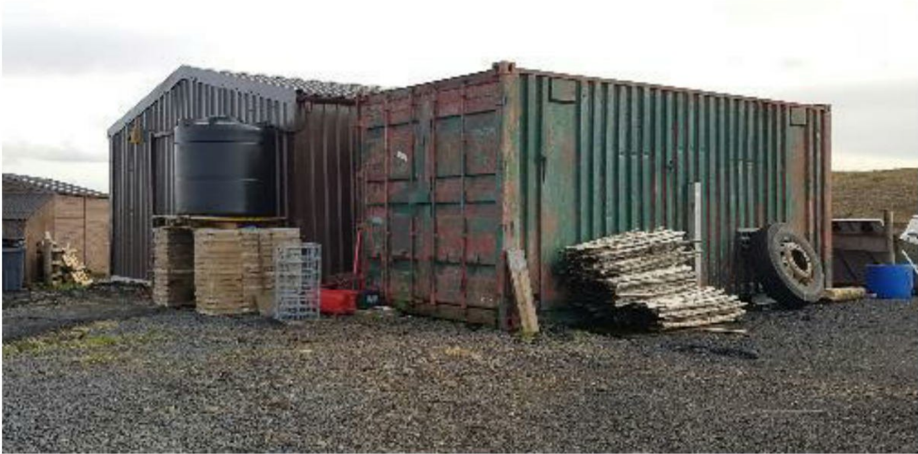
Photograph 1: Site of proposed new timber building
