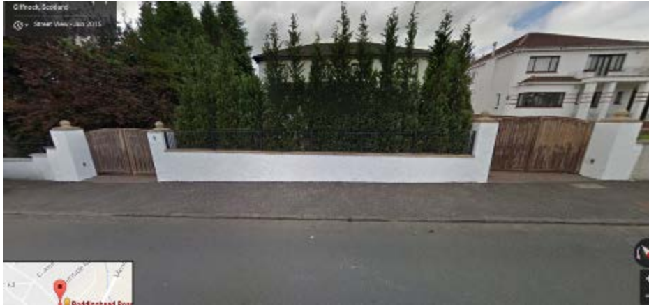
Fig11: Existing Access Arrangement on Roddinghead Road (© Google)
