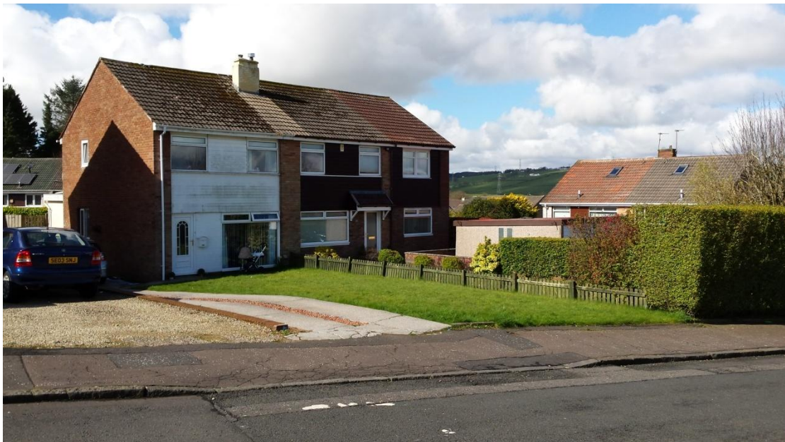
50 Double Hedges with the house with a large gable extension almost doubling size of existing house and roof following existing pitch
