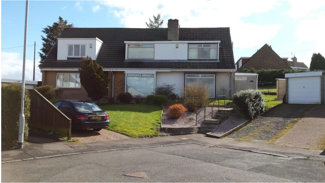
43 Double Hedges with the house doubled in size with roofline following existing pitch
