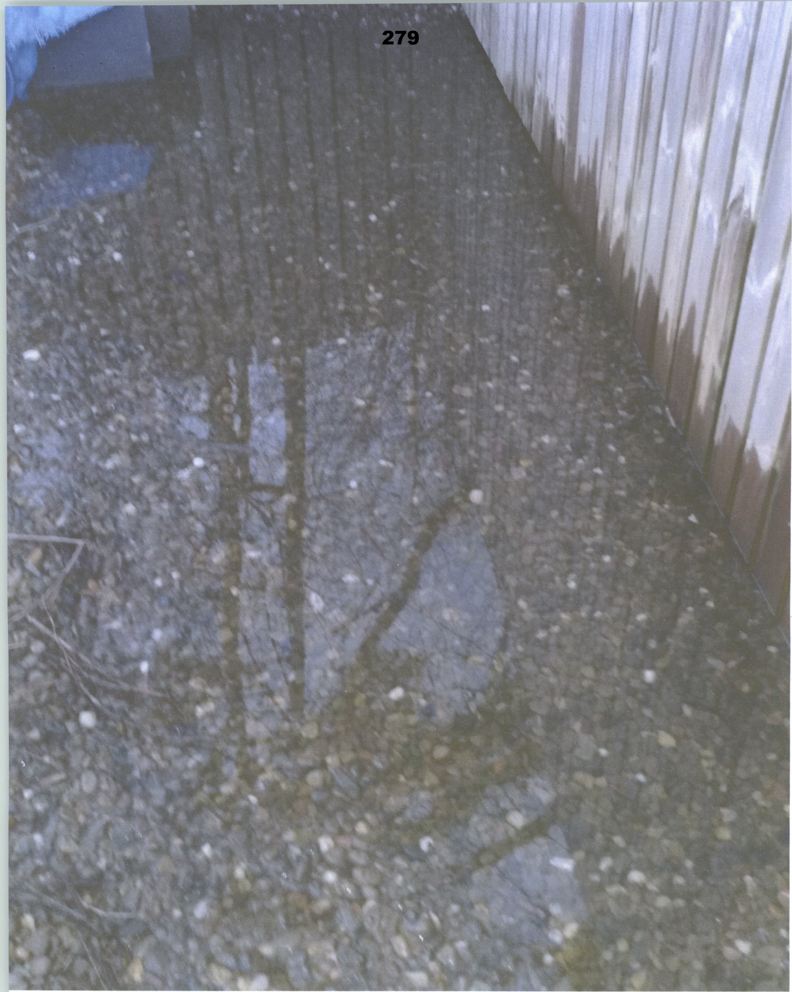
WATER RETENTION IN GARDEN OF PLOT 4
