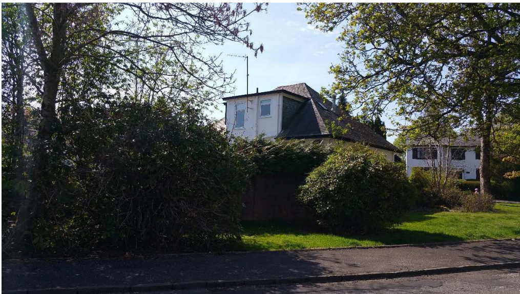
Application site with open space to North and East.
