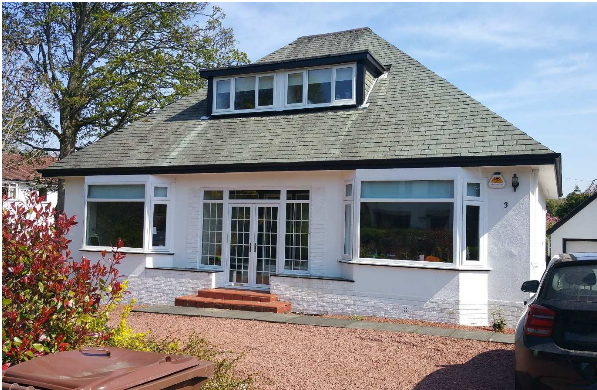
Application site front elevation
