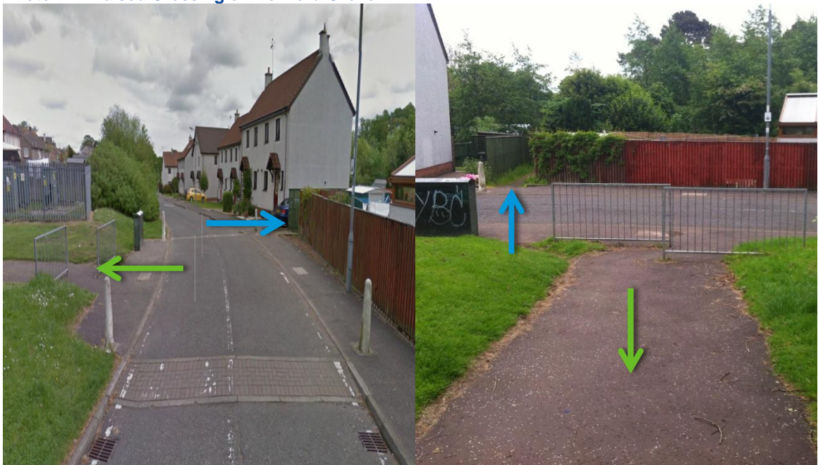
Photo 4-2: Raised Crossing on Newford Grove
