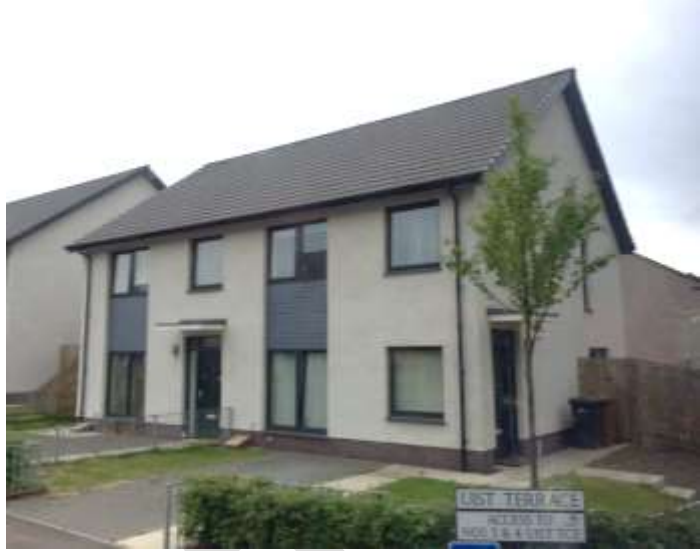
This semi-detached house in Dundee has frontage to two different roads addressing its corner location.
