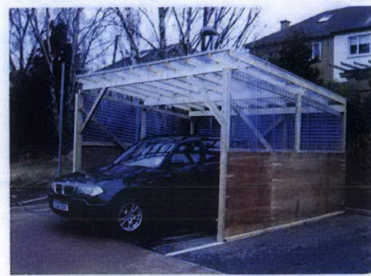
Oblique view of built Valeting Shelter demonstrating that only one car will be valeted at any one time. Ply panel to be finished with Motor Valet Signage.
