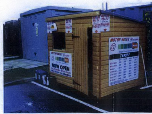
Operation Hut – Pre-fabricated timber panelling, assembled on site. Standard hut base size 2500mm x 1800mm. Car Wash space beside hut.
