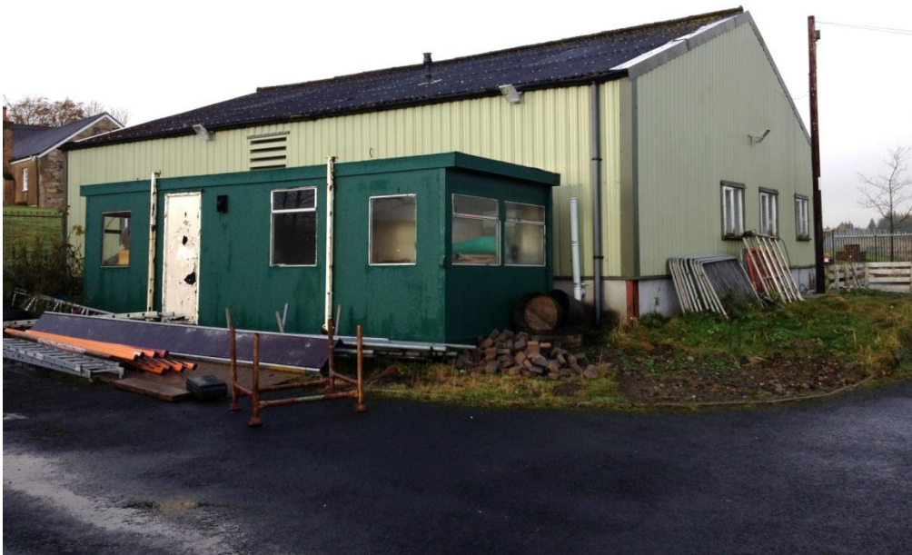
4.5 Side and rear of existing barn viewed from North East
