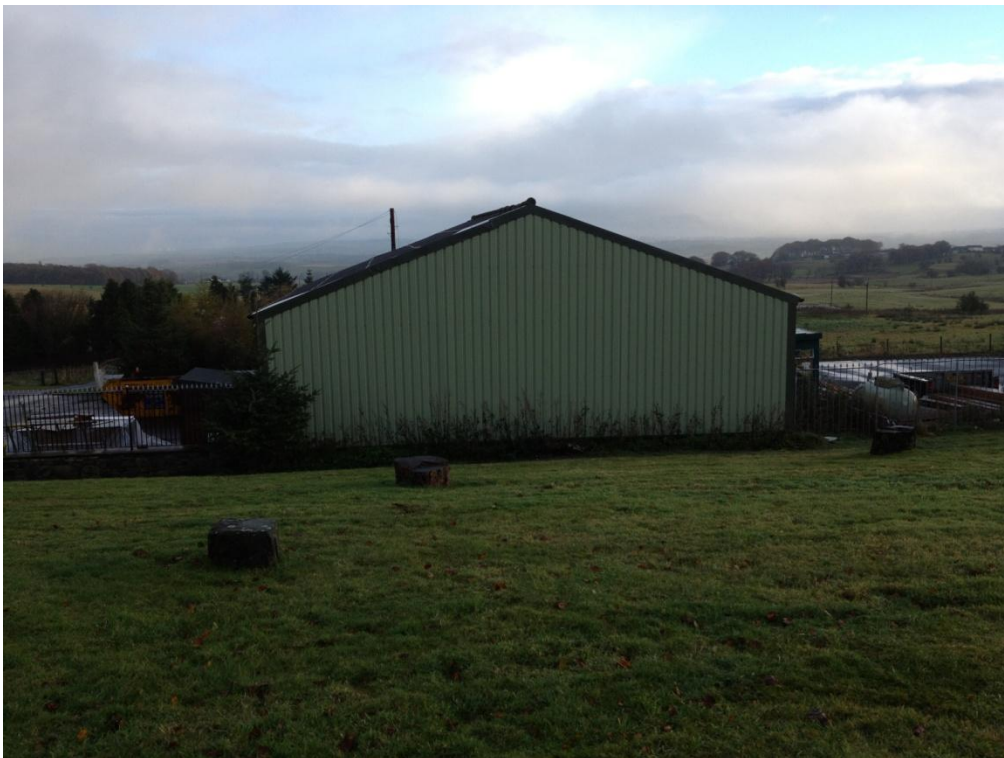
4.3 Existing barn viewed from South West
