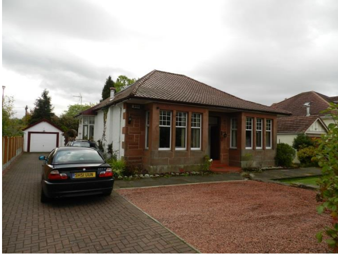
Photo 1 - View of Front of House from Ayr Road
