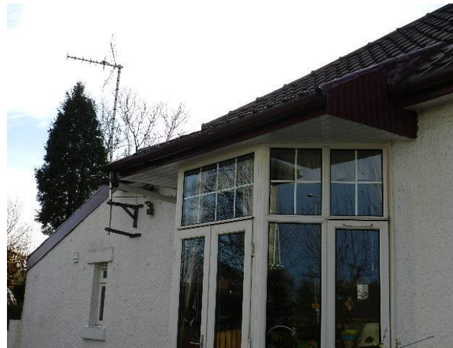
Photo 4 – View of kitchen Roof and bay window roof from Driveway
