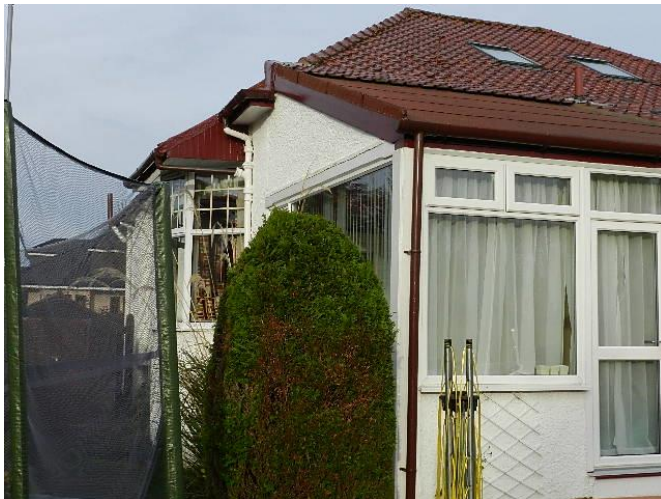
Photo 3 - View of Sunroom Roof at Rear of House
