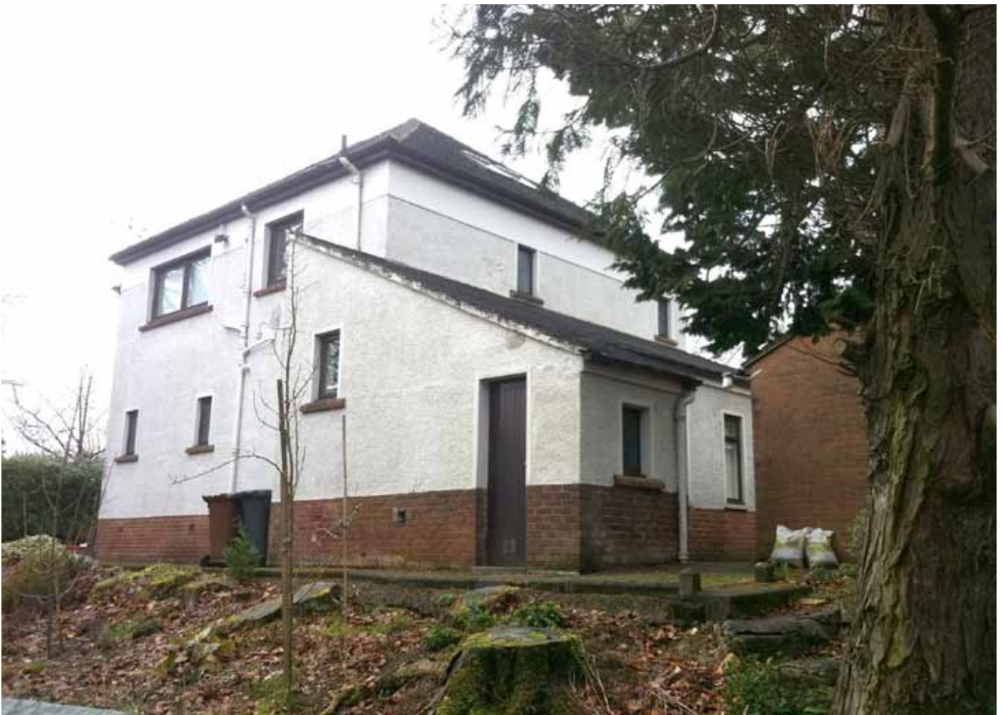
view towards the north east elevation
