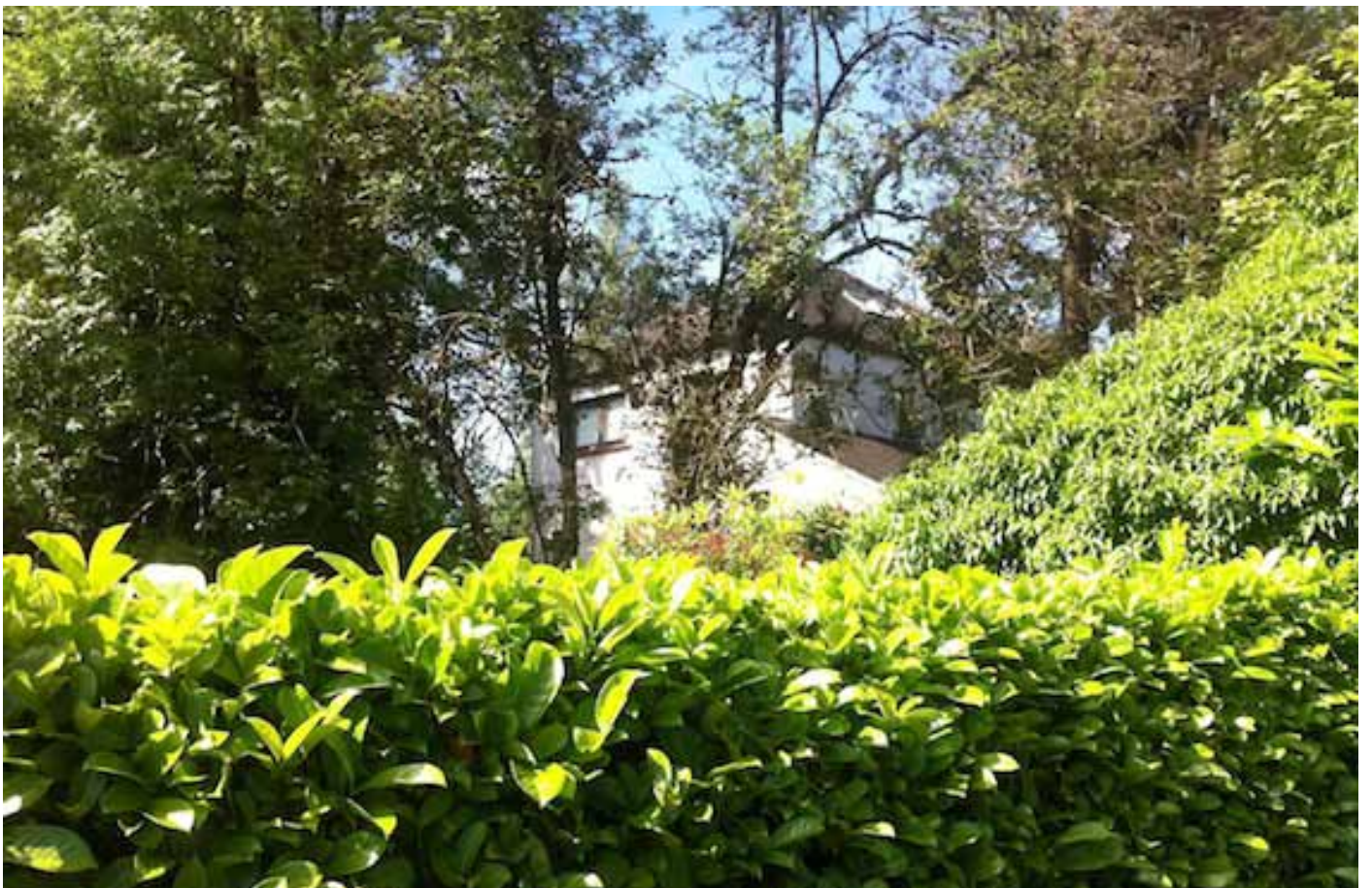
south west elevation from street
