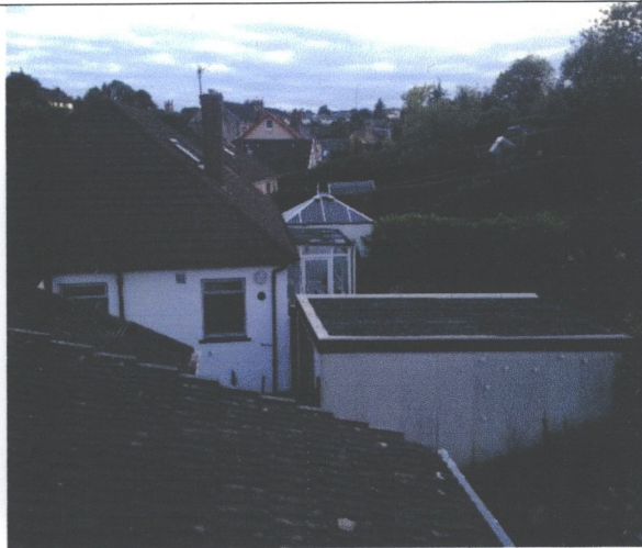
View towards no 25 Viaduct Road from rear. 2 above gutter line Metres
