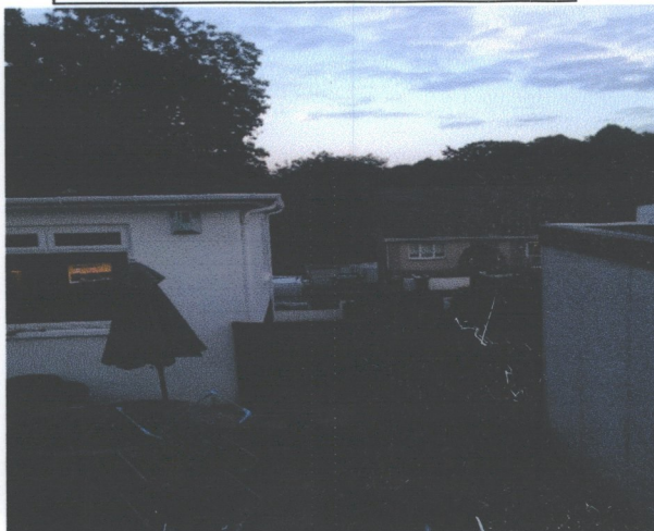
View towards 16 viaduct road. Gable end
