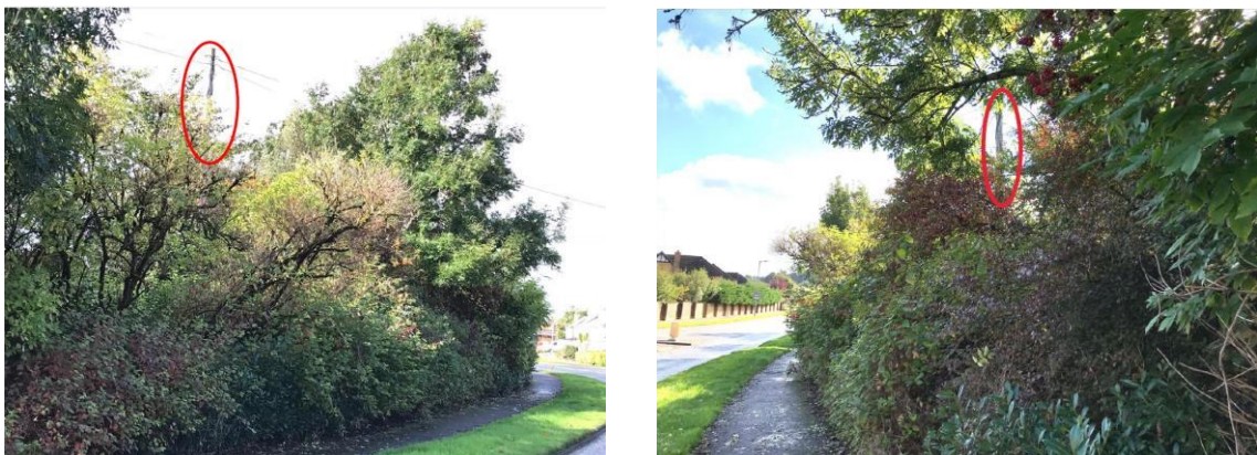
Figure 13: Amenity buffer retained between Barrhead Road and application site (Oct 2021)
