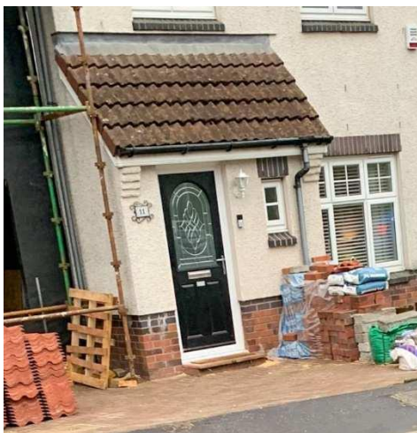
Photo: 11 Kiloran Grove, Application No.2020/0727/TP.
