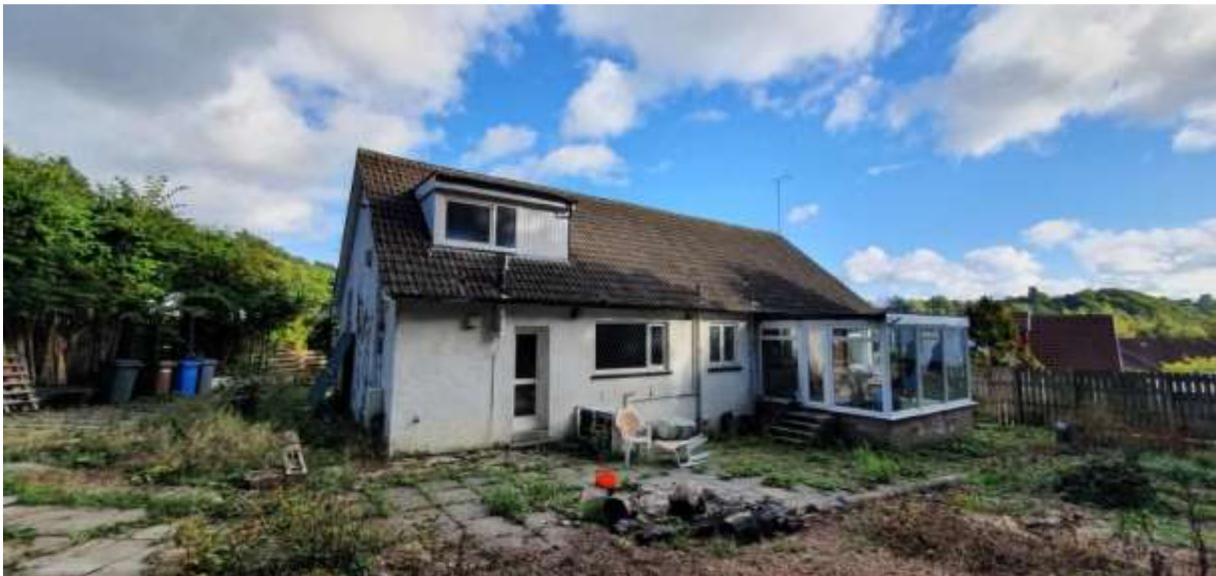
Plate 2. Rear of building
