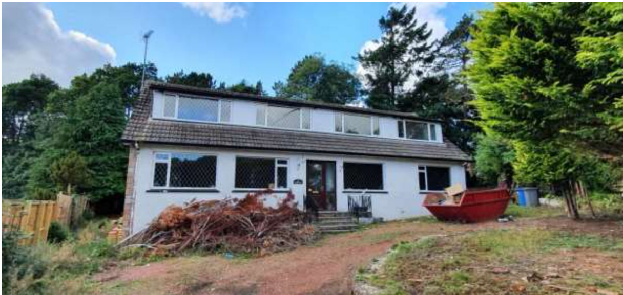
Plate 1. Frontage of Building
