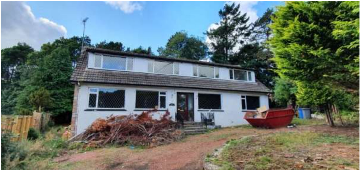
Plate 1. Frontage of Building
