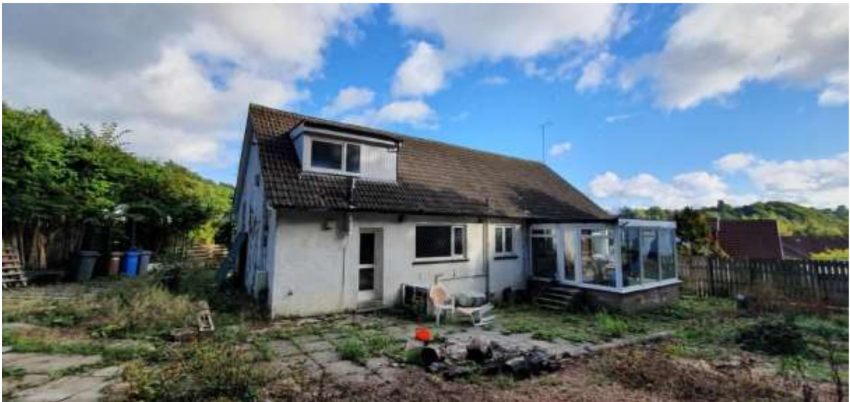
Plate 2. Rear of building
