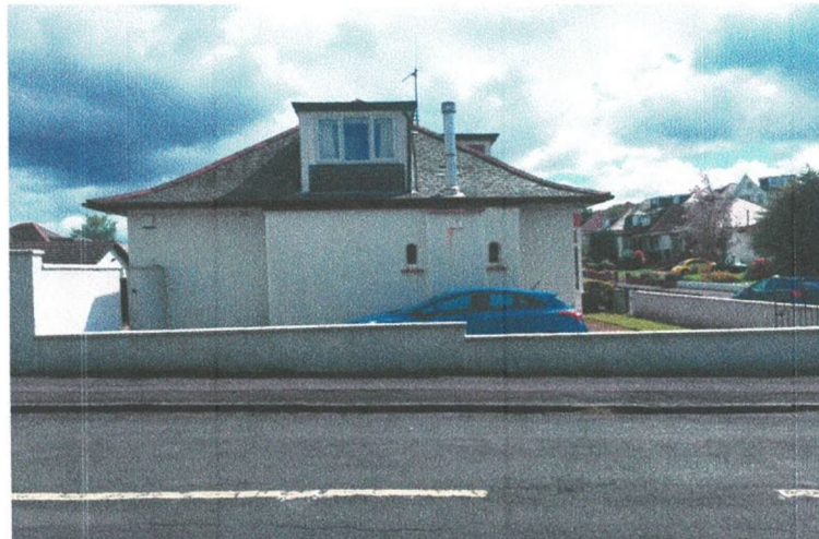
Existing house...side facing Leabank Drive
