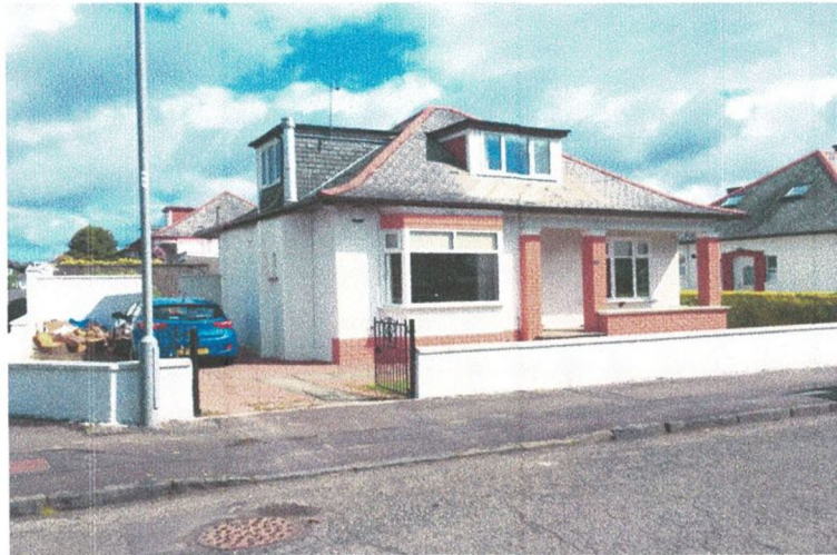
Existing house...front facing Netherlee Road
