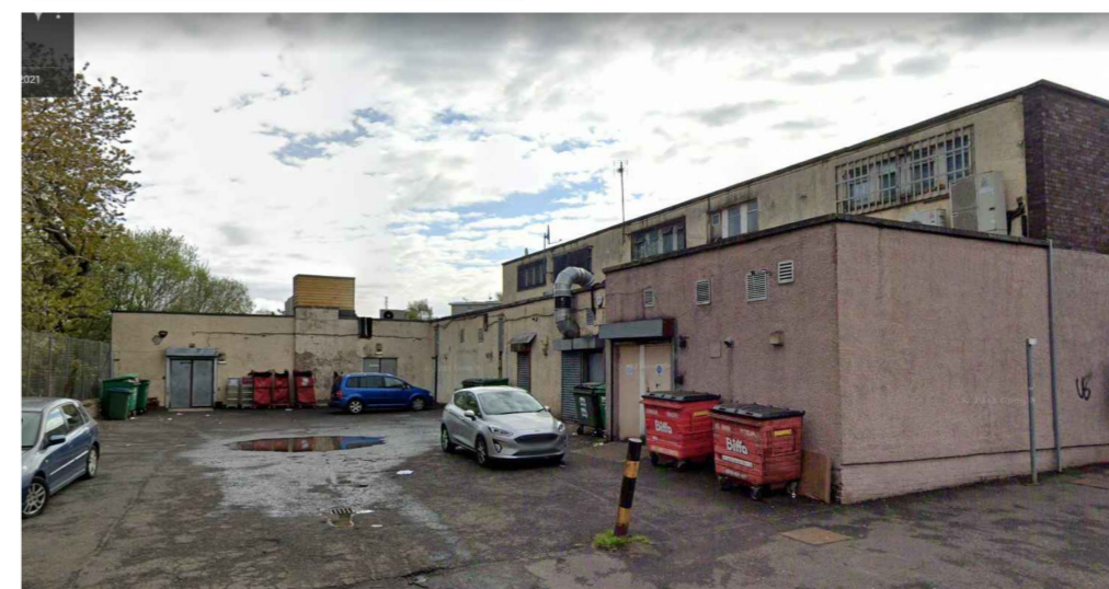
PHOTO OF REAR ELEVATION
