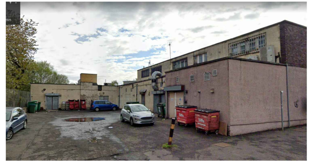
PHOTO OF REAR ELEVATION
