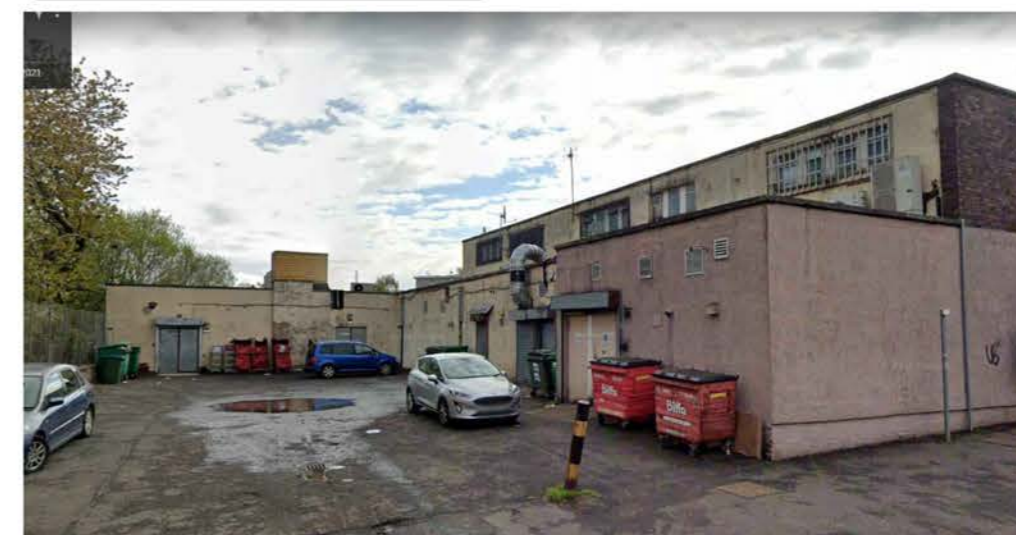
PHOTO OF REAR ELEVATION
