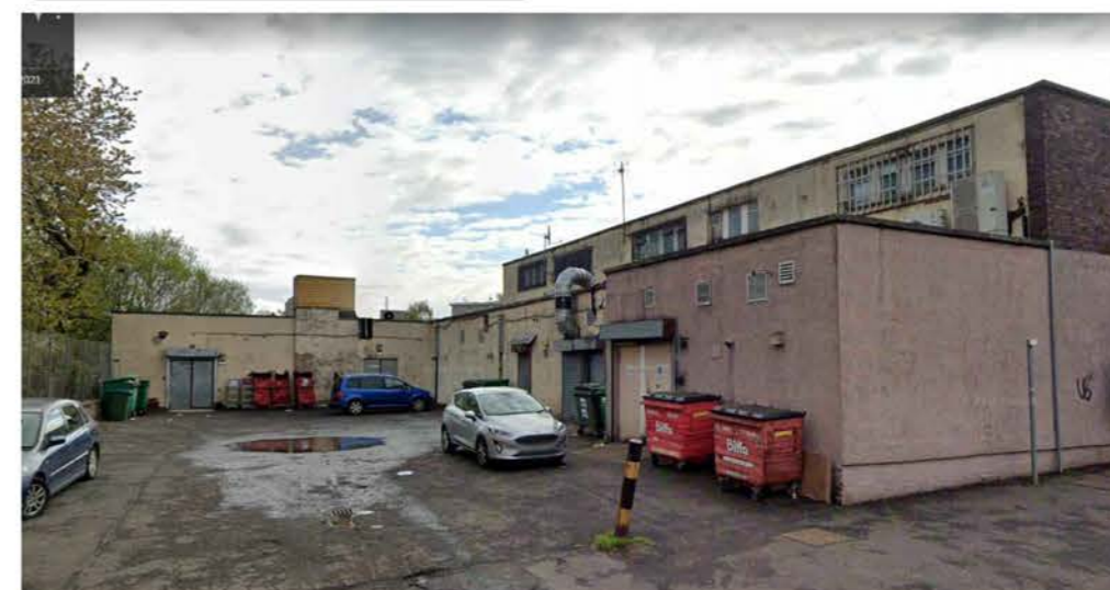
PHOTO OF REAR ELEVATION
