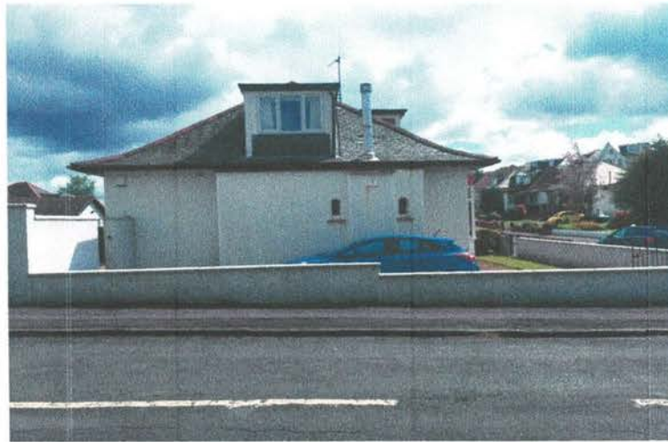
Existing house...side facing Leabank Drive
