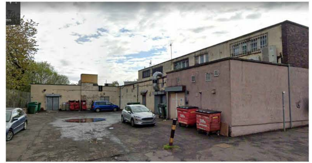
PHOTO OF REAR ELEVATION
