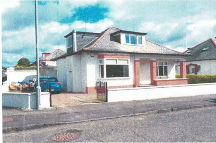
Existing house...front facing Netherlee Road
