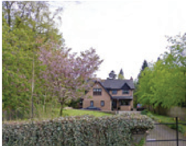
12. Recent development on Springfield Road
