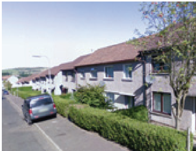
4. Divernia Way looking west
