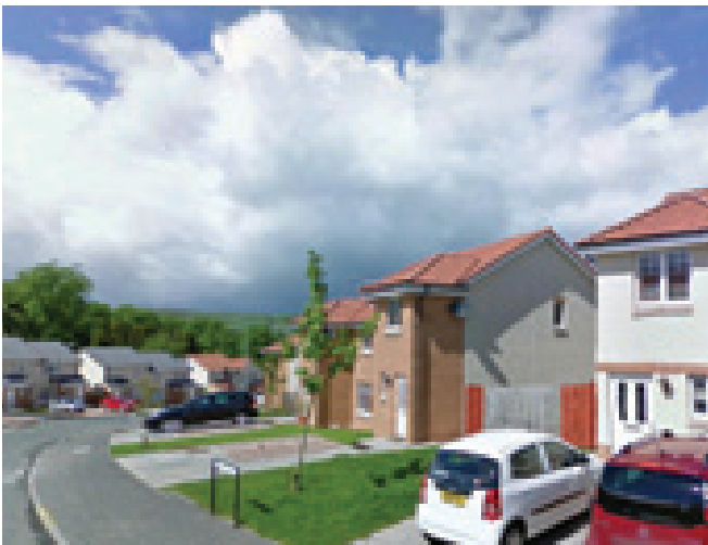
8. Recent development on Divernia Way looking west
