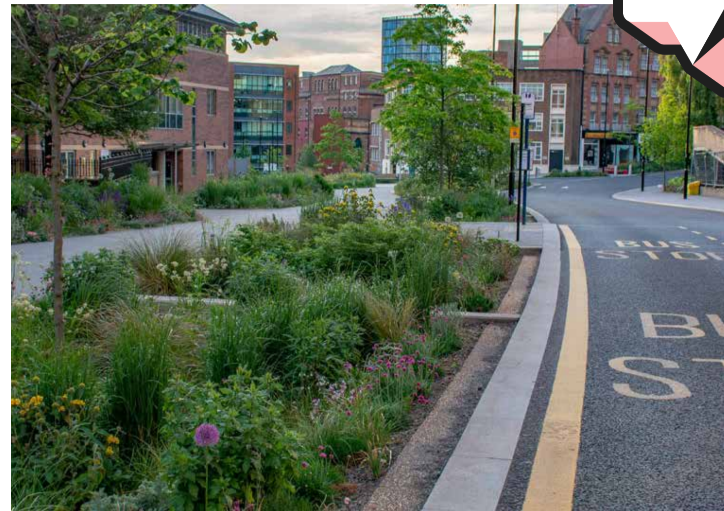
The 'Grey-to-Green' project in Sheffield showcases how roadside rain gardens can be used to successfully improve drainage, biodiversity, and critically, community placemaking. A case study on the scheme shows an on-balance reduction in maintenance costs.
