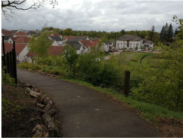
New path constructed by Cala Homes
