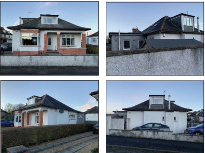
03 Existing Photos Scale NTS @ A1
